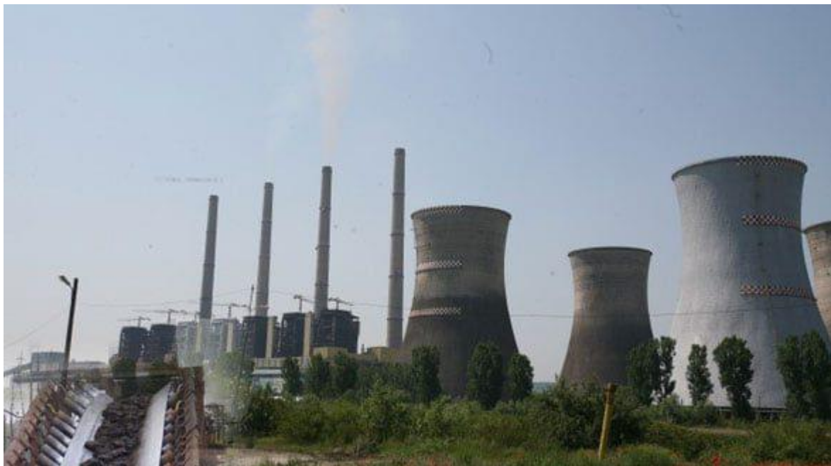
Figure The Turceni thermal power plant.
